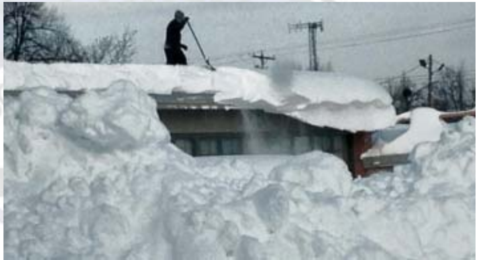
Clearing snow off of the school roof.
